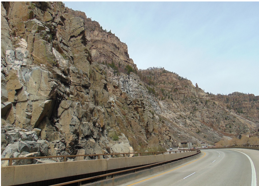
Figure 4. I-70 Glenwood Canyon MP 124
