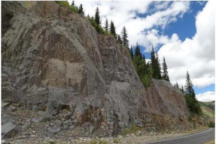
Draped mesh and bolts
