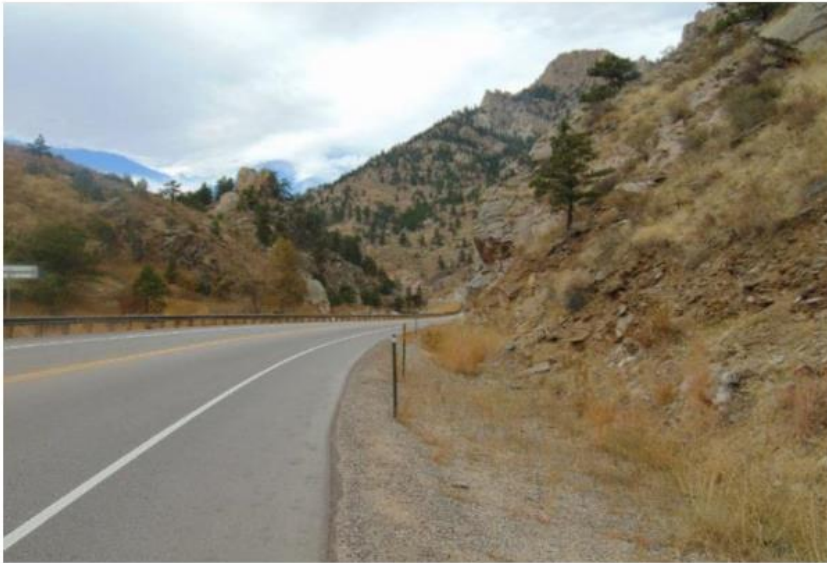
Westbound viewshed, cut in center right, across from treed slope
