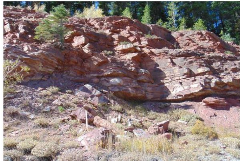
Sandstone undercut by weaker shale; boulders at base of cut
