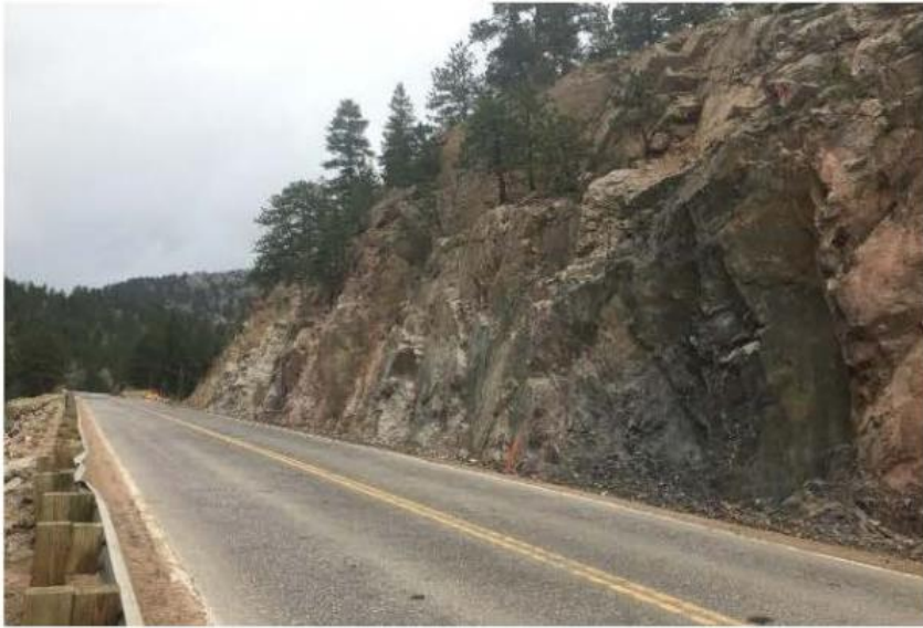
Vegetated benches in cut, view to north
