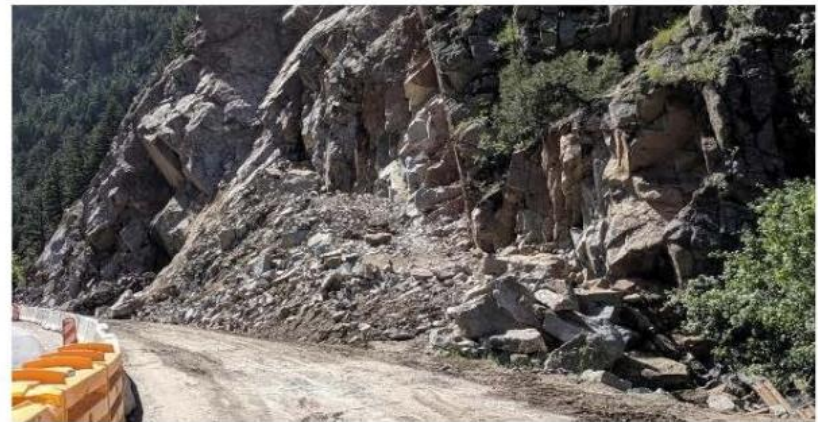
Cut slope early construction view to SSE
