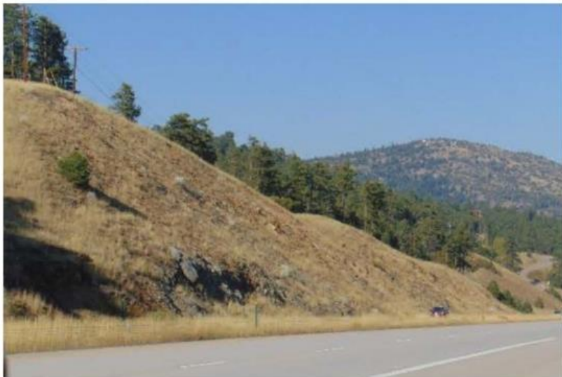
Cut slope mixed soil above rock
