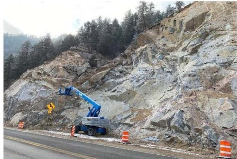
Cut slope post construction view to SSE
