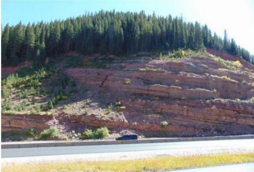
Terraced, bench slopes with revegetation
