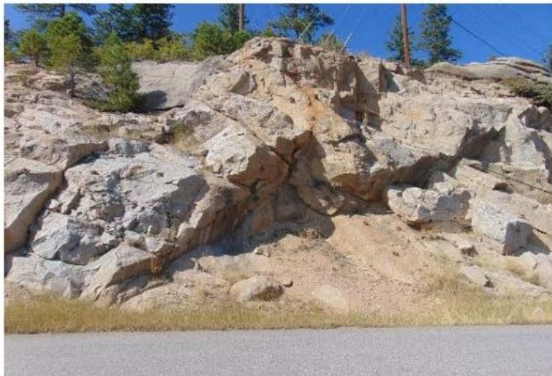
Rockfall mitigation, shotcrete, bolts
