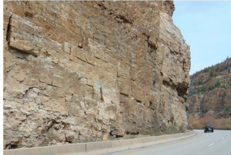
View to northeast from eastbound lane
