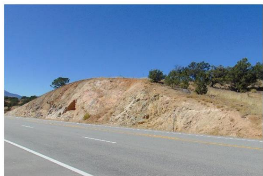
View to west-southwest, cut without mesh with angular gap
