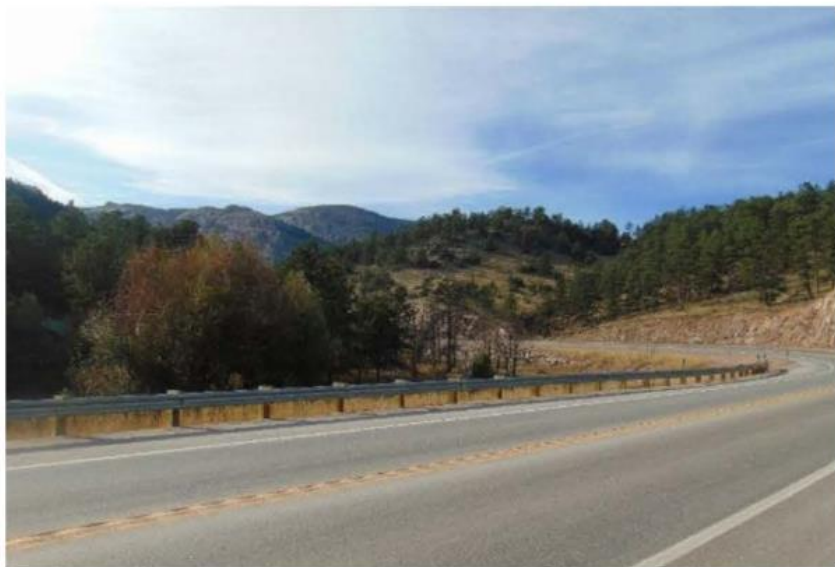
Westbound viewshed, cut around curve left (west) of drainage
