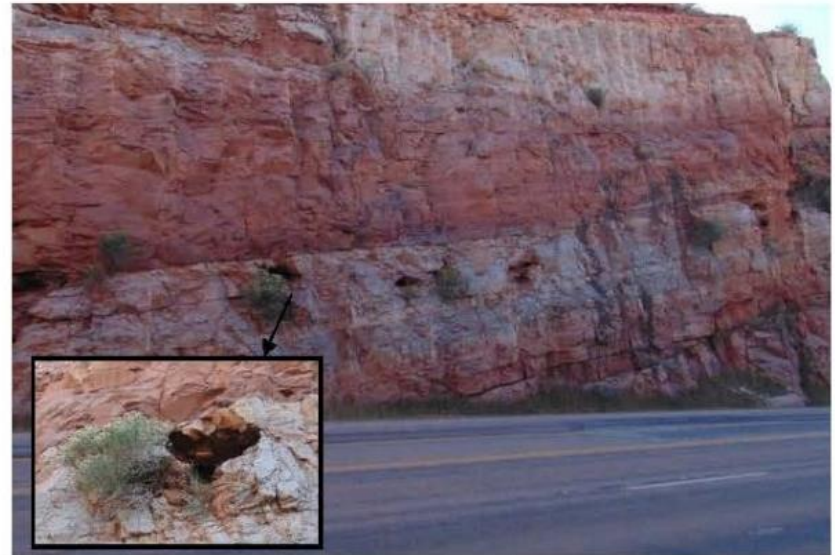
Dissolution cavities and boulders in ditch
