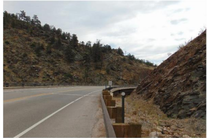
Eastbound view, cut is center right, left side of road
