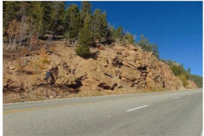
View to northeast, cut east of emergency truck ramp
