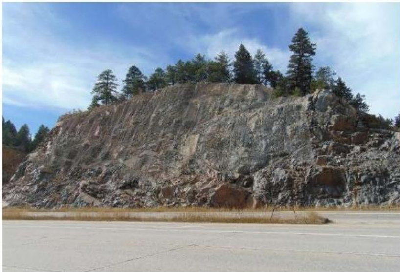
Draped mesh, view to northwest
