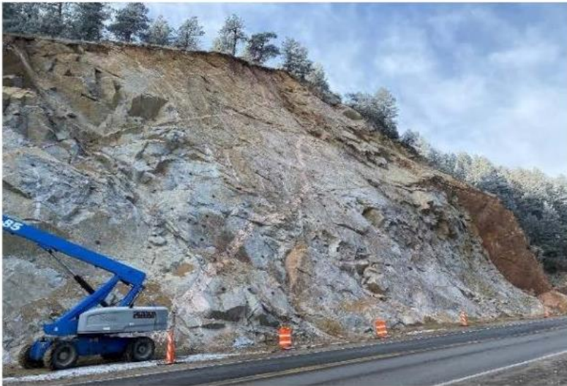
Cut slope post construction view to west
