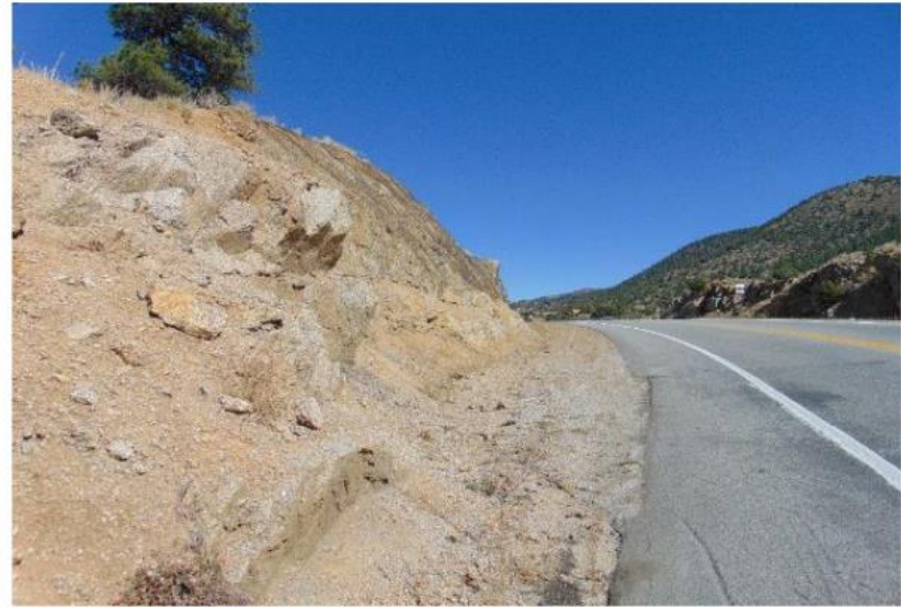
View to north-northeast, rock mesh and catchment ditch
