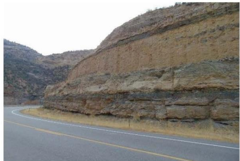
View to SE, middle area of cut
