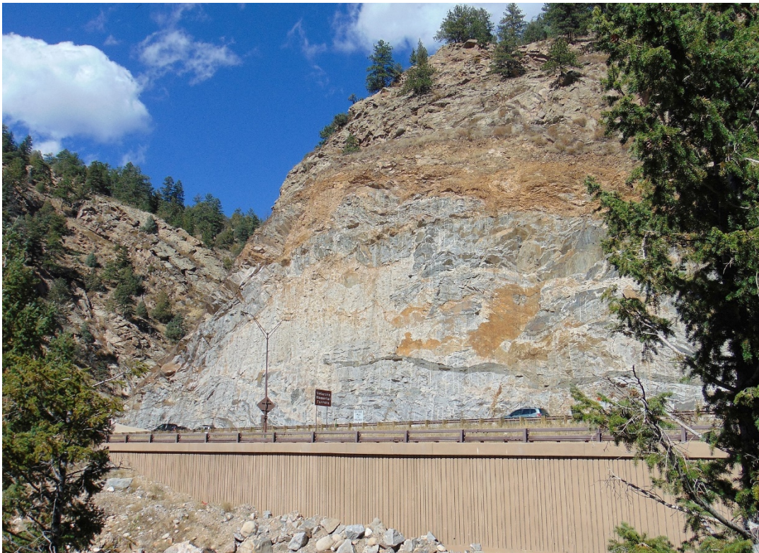
Figure 7. I-70 MP 242, Veterans Memorial Tunnels
