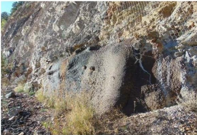
Drains in cut
