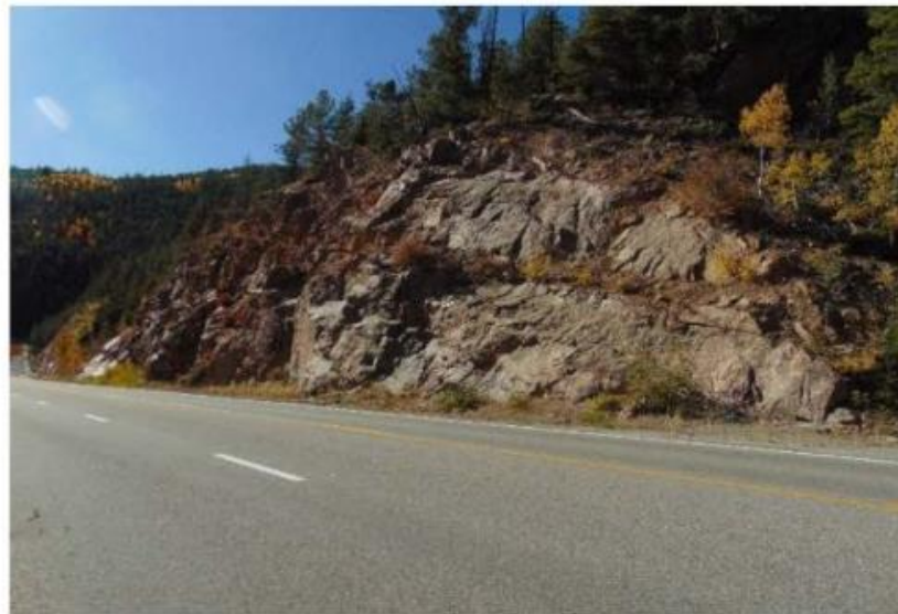
View to southwest, benches with vegetation, emergency truck ramp on left
