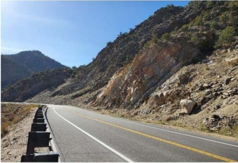
Eastbound View, looking southeast at east end of cut
