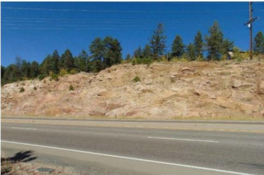
Cut, looking north
