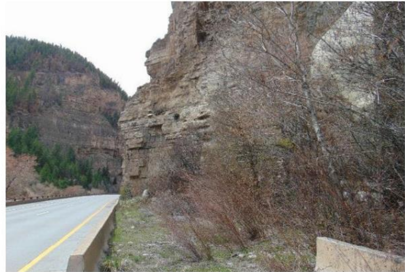
View to west-southwest; little to no ditch area behind barrier
