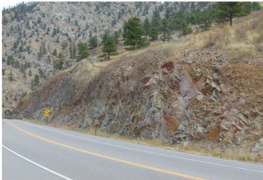
View to north-northwest, anchors at top of cut, draped mesh
