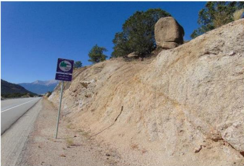
Machine marks in cut below perched boulder
