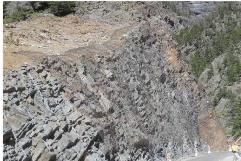
Installation of mesh in 2011, view southbound
