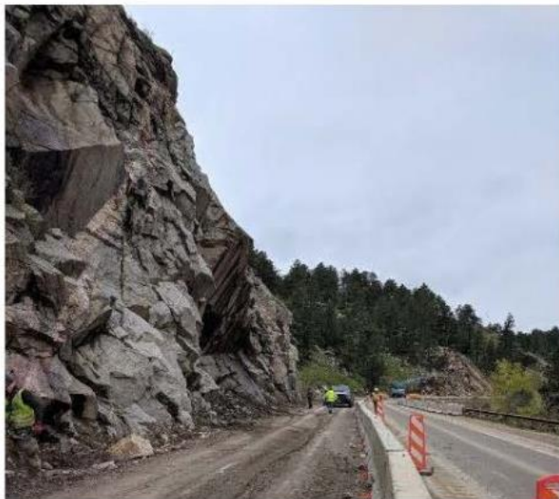
Cut slope early construction view to WNW
