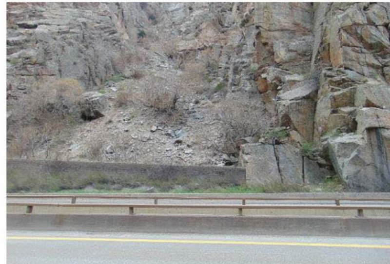
Wall at northeast end of cut, looking west
