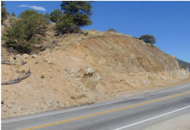
View to northeast, rock mesh
