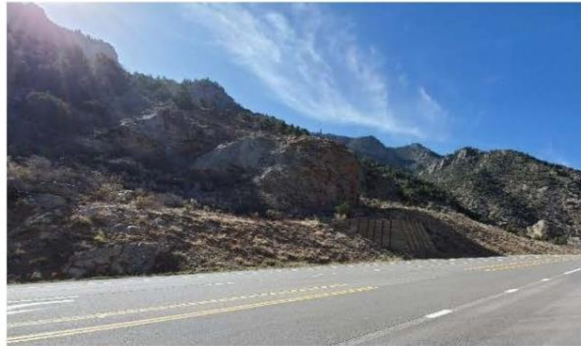
Structure east end of cut, looking south-southwest
