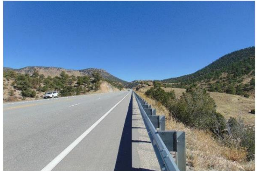
Eastbound viewshed, cut is center left of road
