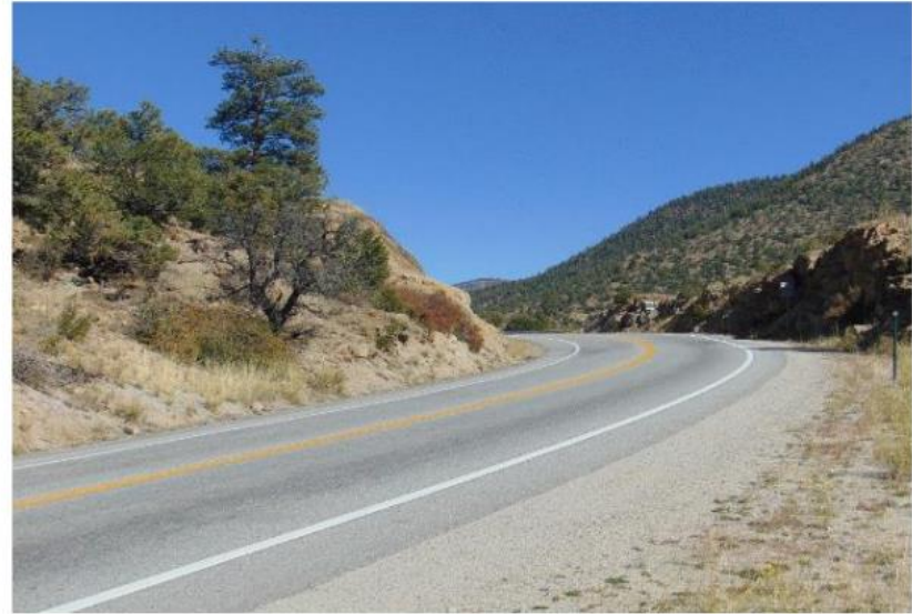
Eastbound viewshed, center left beyond brown shrubs
