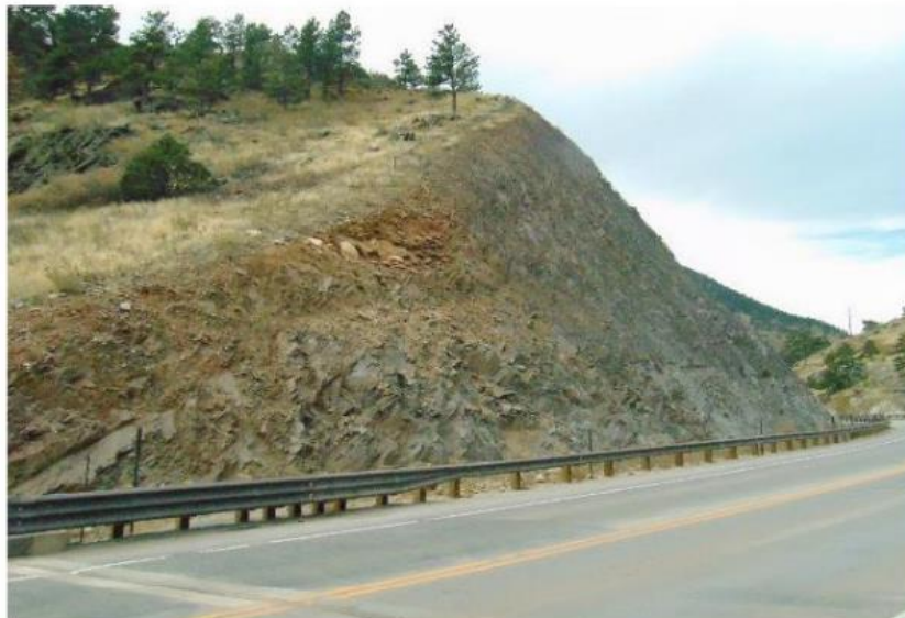
View to southwest, anchors at top of cut, draped mesh
