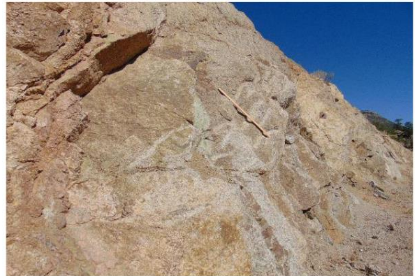
View to northeast with machine marks, bolt
