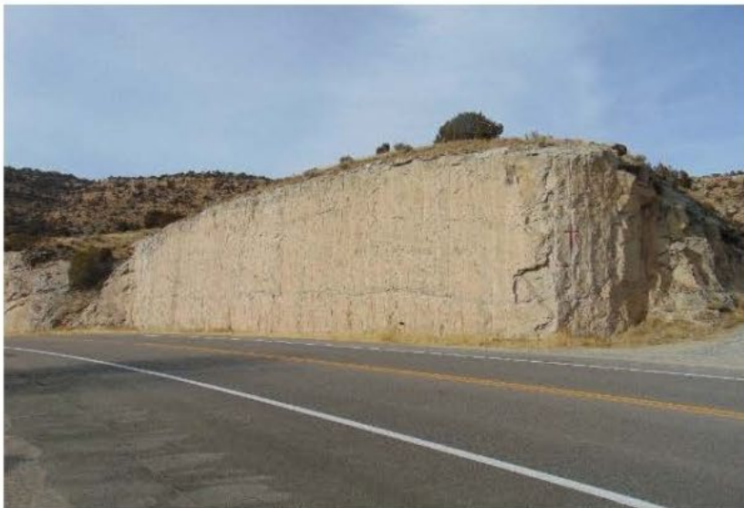
NW view of two different blast techniques (far left of photo and center)
