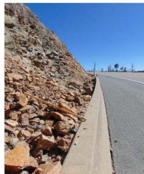
Rock filling behind barrier
