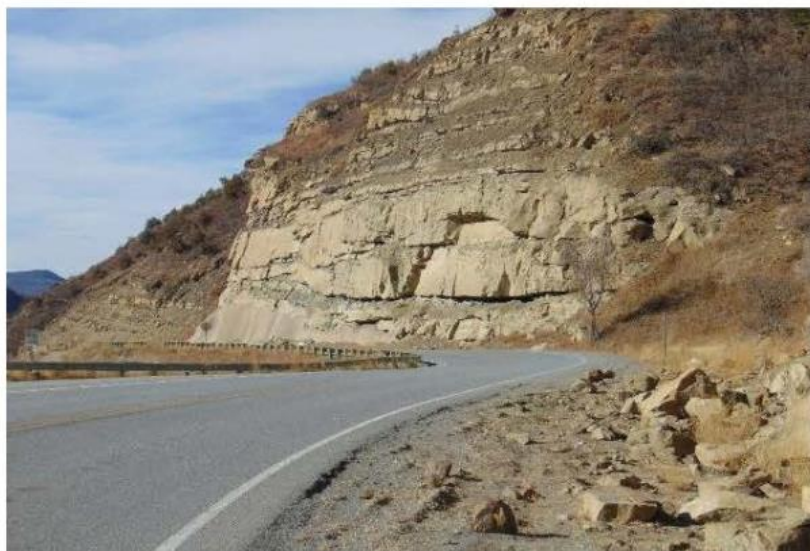
View to west, undercut sandstone, shotcrete lower slope
