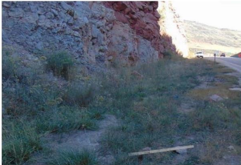
Change in rock type; rocks in ditch with red boulder near face of cut
