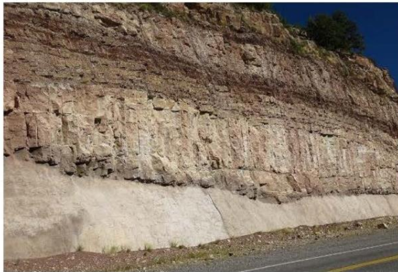
Draped mesh and shotcrete base
