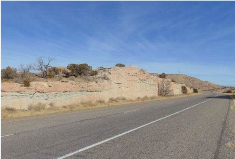
View to northeast
