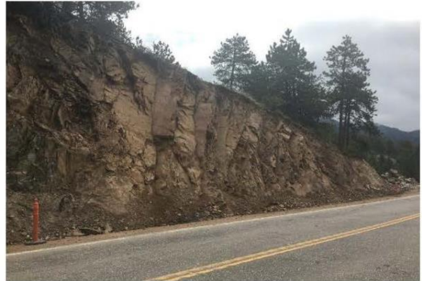
South end of cut, view to east
