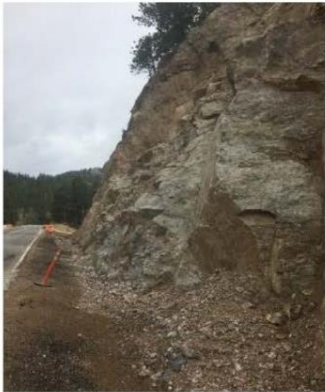
Cobbles at base of cut, view to northwest
