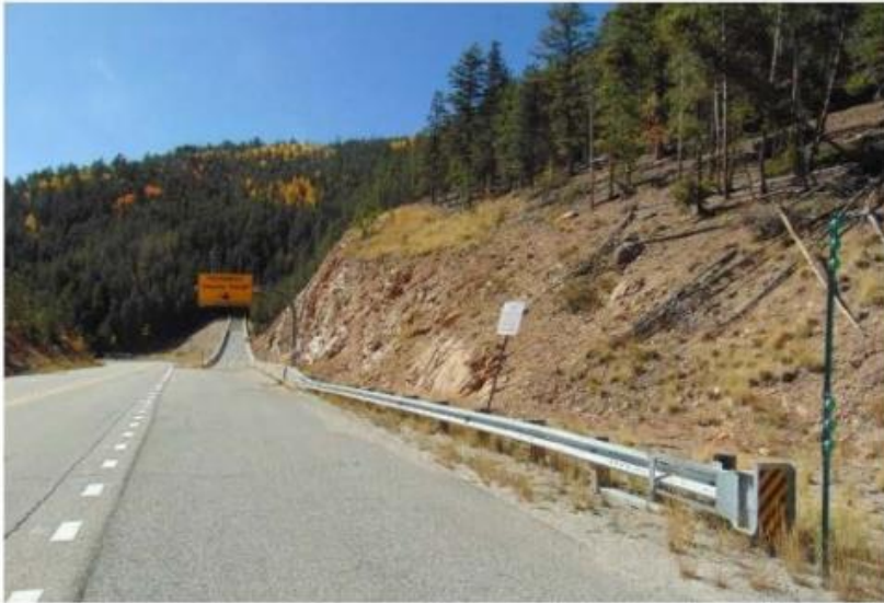
Westbound viewshed, view to west-southwest
