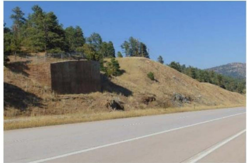
Eastbound viewshed with upslope wall
