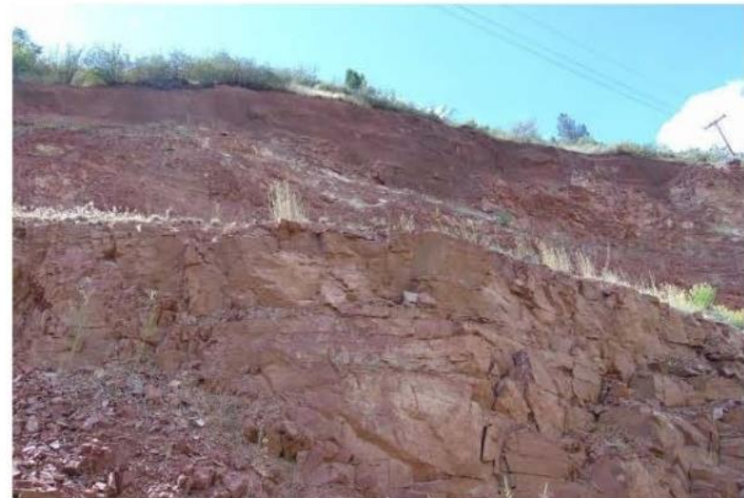
Shotcrete at top of cut
