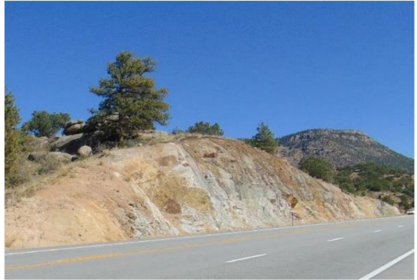
View to northeast, draped mesh at west end
