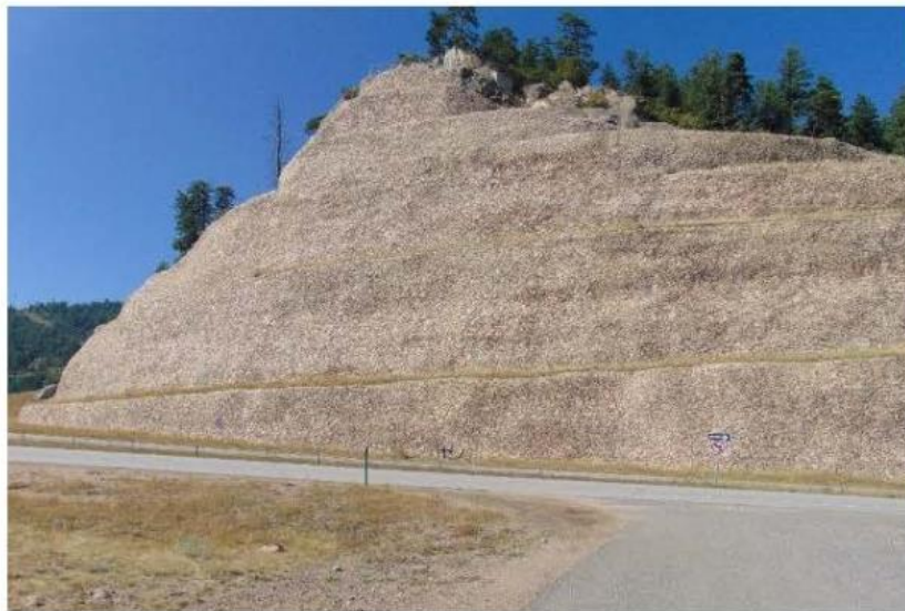
Cut area with terraces and rock facing
