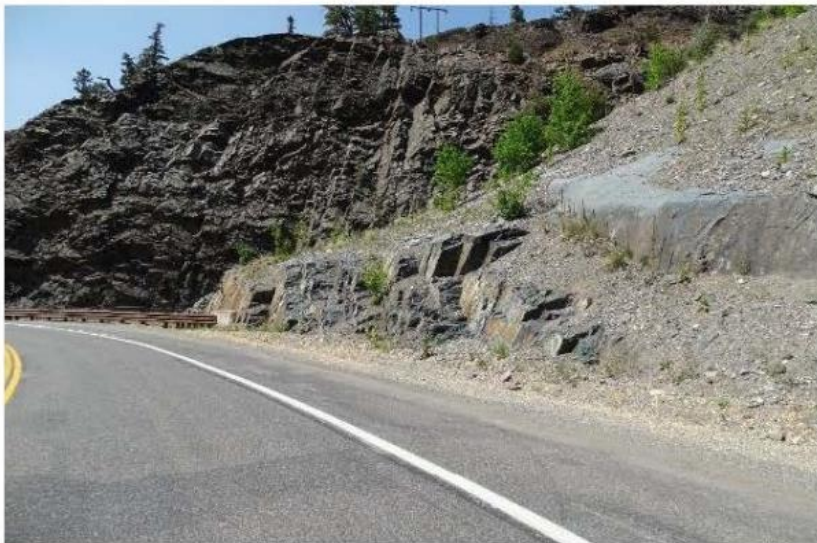
Terraces and adjacent cut northbound
