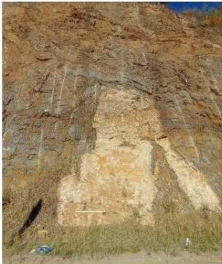
Draped mesh over half cast blast features
