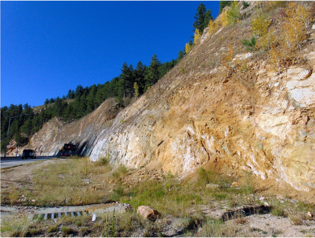
Figure 8. SH 119 MP 6 Catchment Ditch
