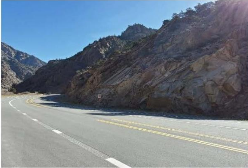
Eastbound View, looking northeast
