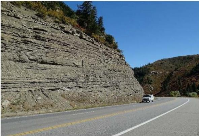
Rock and sediment debris at base of slope
