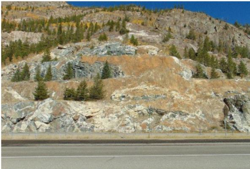
Cut view to northwest of vegetated, terraced slope and iron staining
