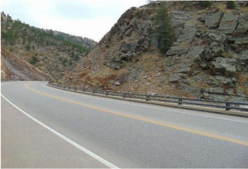
Eastbound viewshed, cut on right (south) side of road at curve
