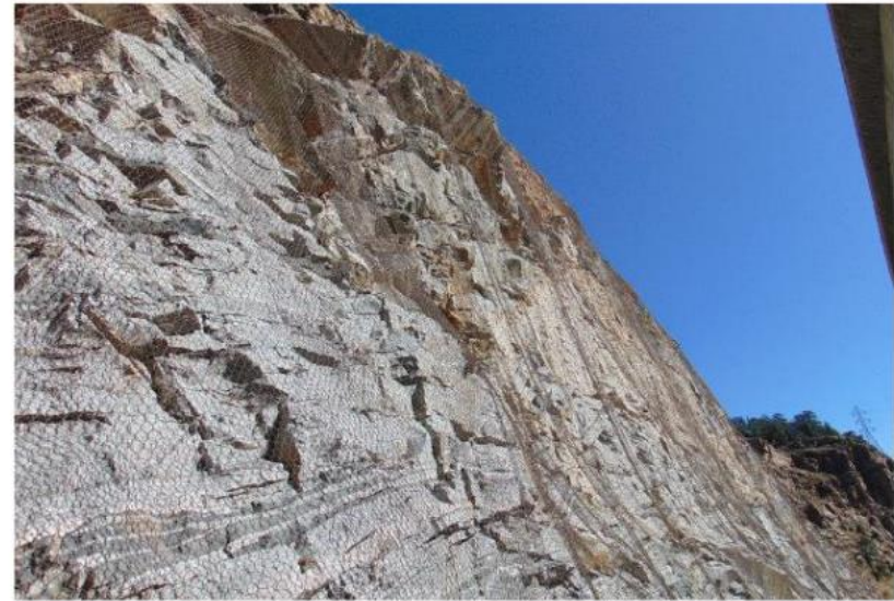
View to northeast, mesh, bolts
