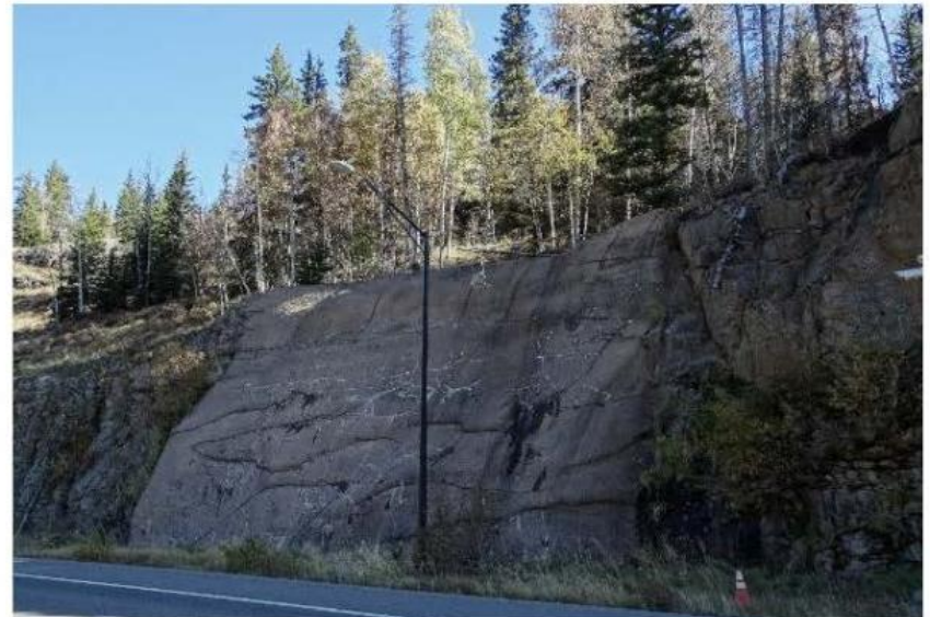
Shotcrete south of west portal
